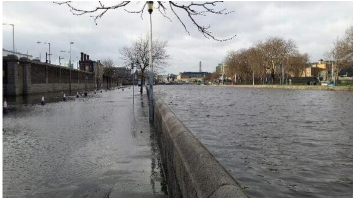
Figure 4: Flooding at Victoria Quay in January 2014
